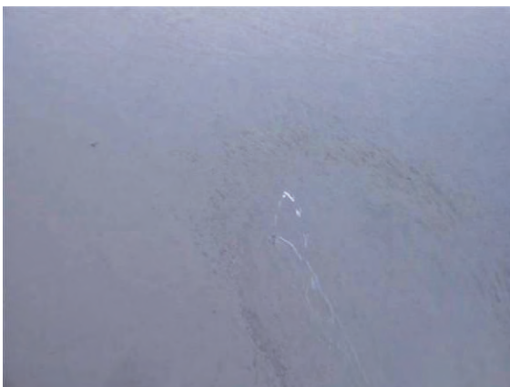
Figure 5. Photos show examples of Class III leak
